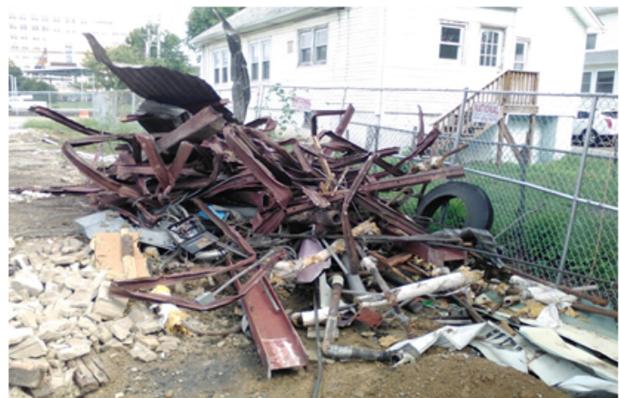
Steel debris separated for recycling.
