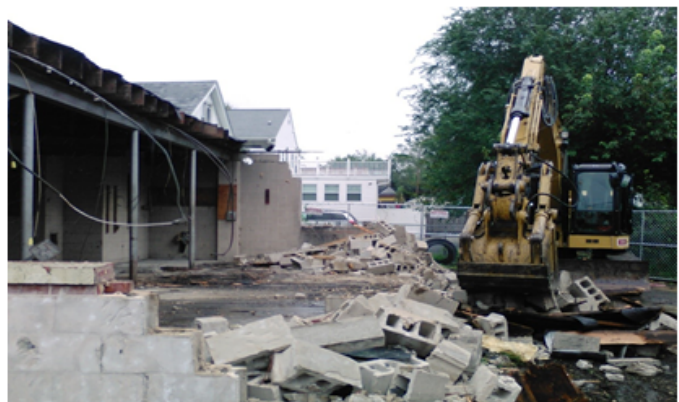
Debris staged at rear of building to load in roll-off containers.
